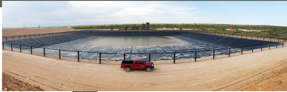
Seely Recycling Containment Pond
